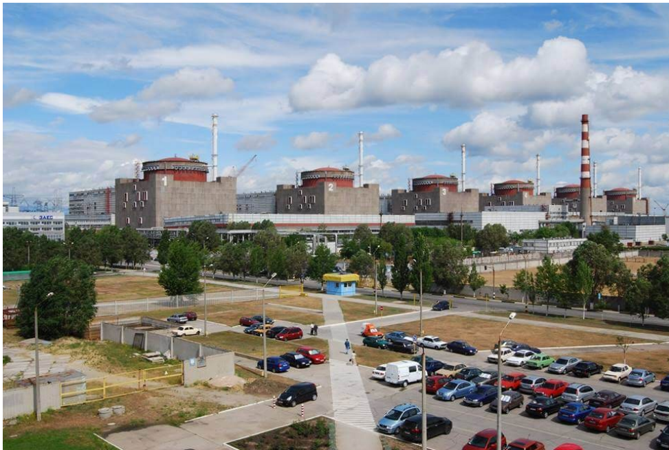
Figure 3: Zaporizhzhia nuclear power plant, Ukraine
